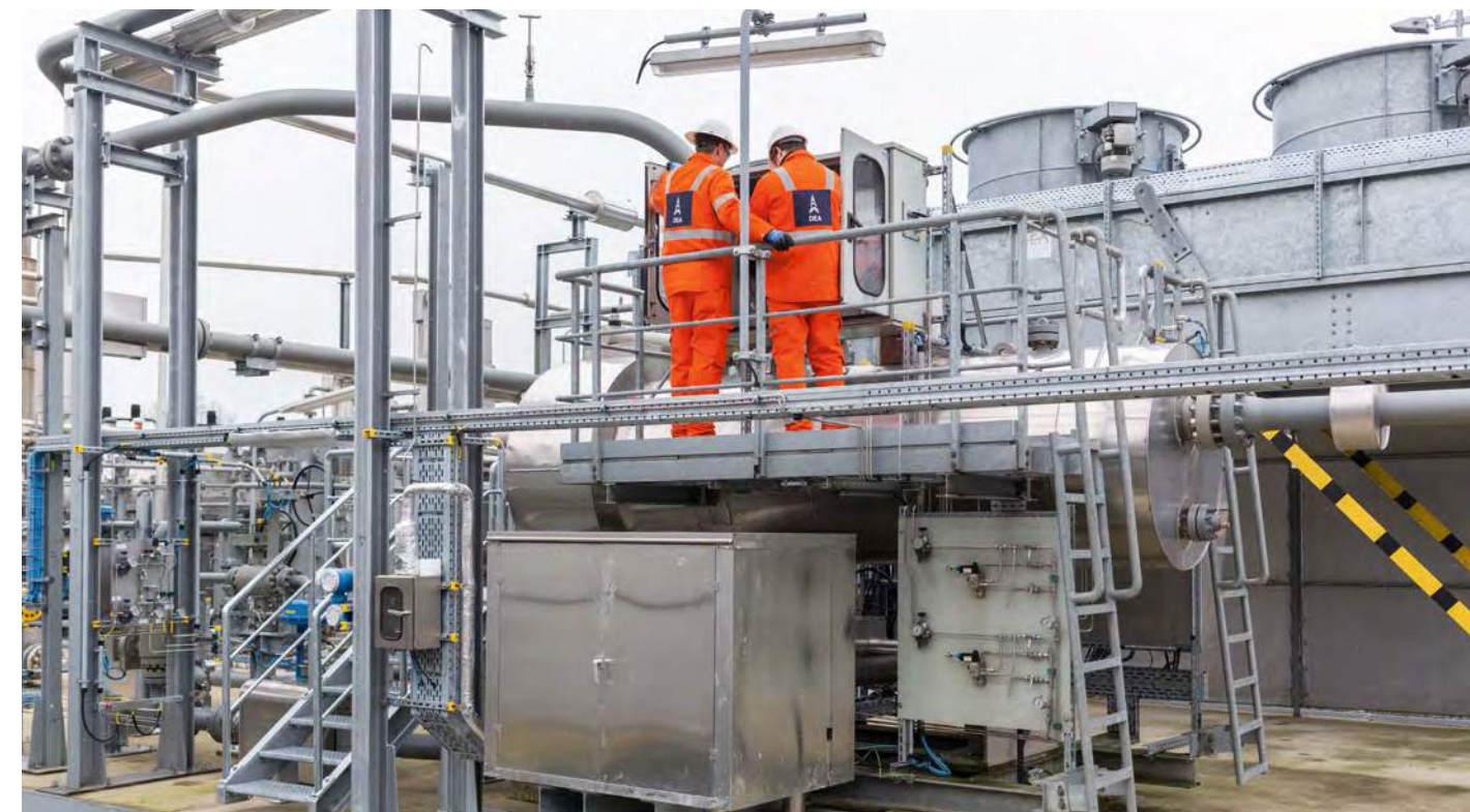
Checking a gas dehydration unit at the Völkersen field
