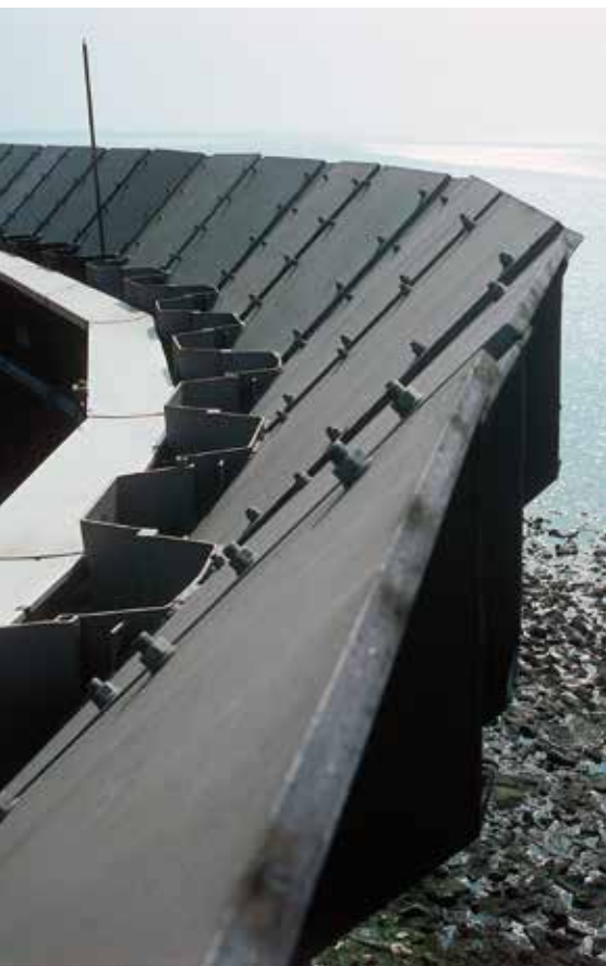
Top: Sheet pile wall with wave deflector. The sheet pile wall facing the open sea extends to a height of 11 meters. Nothing can enter from the outside, apart from rain and spray. And nothing can escape to the outside, not even rain water.
