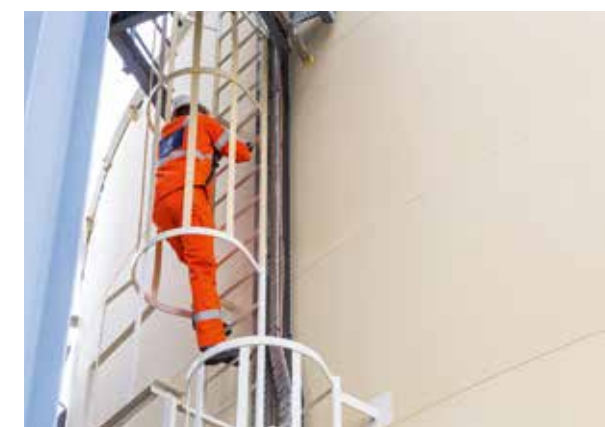
Right: The double-walled oil storage tank for the intermediate storage of the extracted crude has a capacity of 2,000 cubic metres. In the event of damage to the inner wall, the outer hull would safely contain the entire volume of oil.
